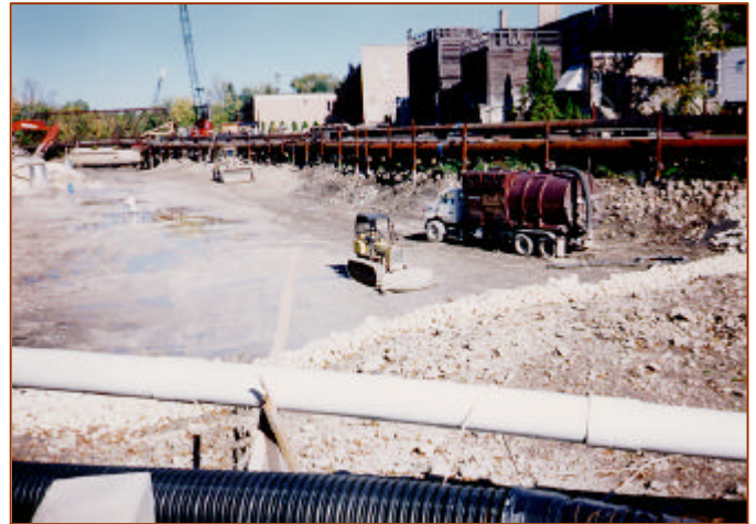
Dry Excavation Activities
