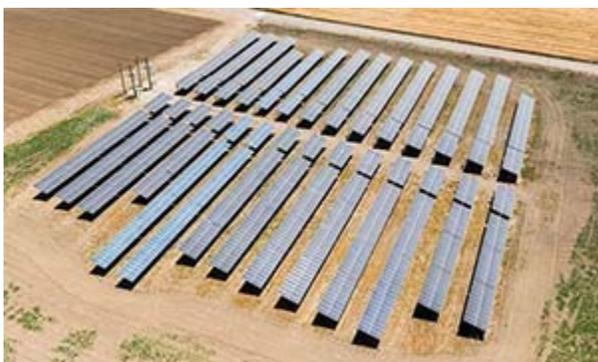
*In the first year of operation, a 792-kW solar system installed on a block of fallow, unusable land at fruit and vegetable grower Uesugi Farms in California generated over \$100,000 in savings and has offset the farm's electric bill by more than 90 percent. Photo courtesy of Vista Solar.*
