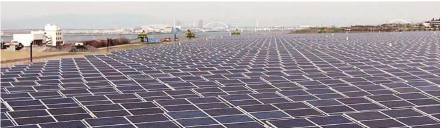
*Hikari-no-Mori, or "Forest of Light," is a mega-solar project of 36,000 solar panels built on top of a landfill on the man-made island of Yumeshima near Osaka and managed by Sumitomo Corp. Photo courtesy of Nissan.*
